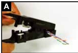
Strip approximate 4cm of the cable jacket.
